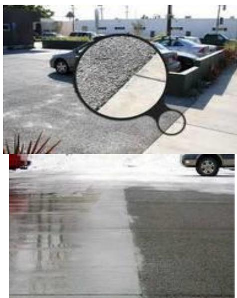
Fig 1.2 Ordinary concrete and pervious pavement
